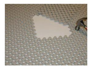
Lagune tiles can be connected easily with a hammer.
